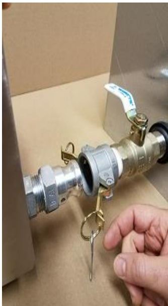
Attach Pump to Valve
